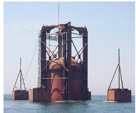
AWS full-scale pilot plant during submergence offshore Portugal, May 2004
