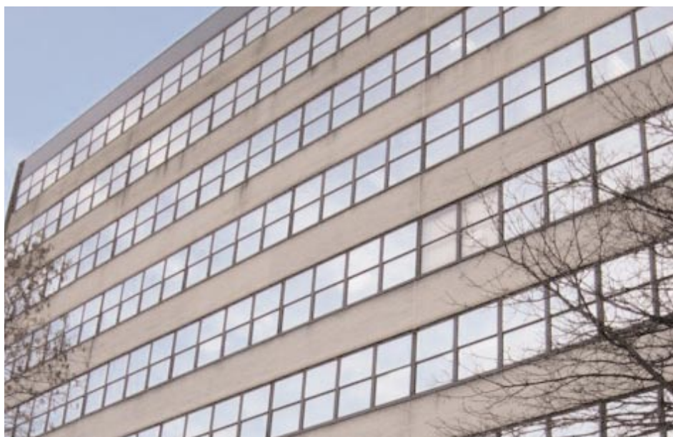
Honeywell House - assessed for viability for economic installation of small scale CHP
